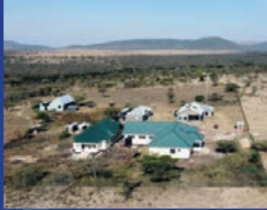
Aerial view of health center
